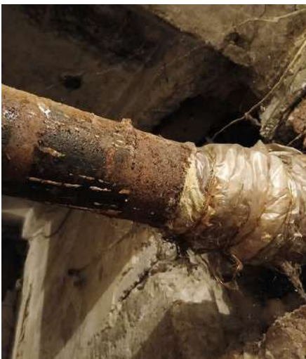
Replacement of sewer risers: 240M
