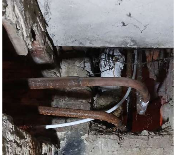
Replacement of water risers: 240M
